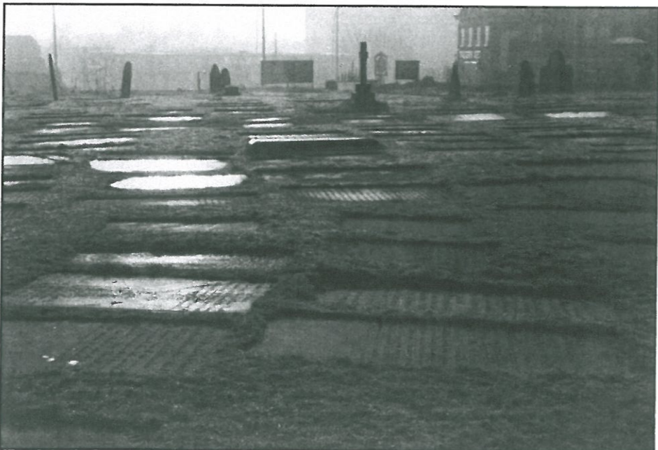
BELOW: Operation groundwork completed.
